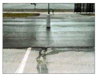
If your asphalt lot or road has cracks or alligatored areas, you need help. Seal the cracks with an Overband Crack Seal and then resurface the entire lot with economical Micro-Slurry Surface.
